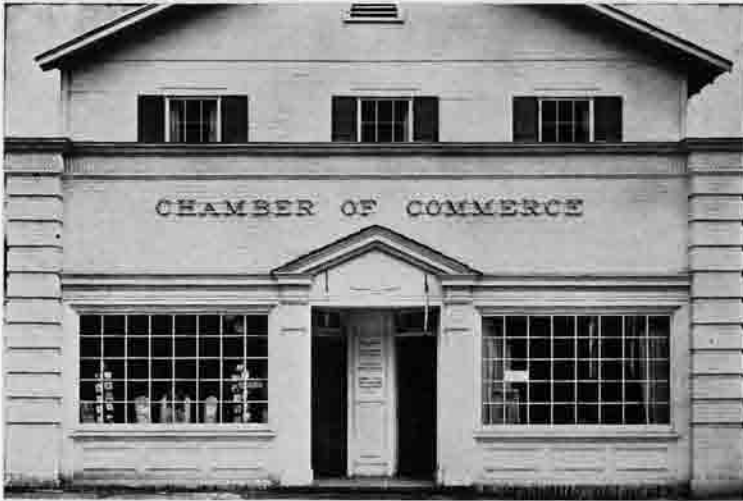
CHAMBER OF COMMERCE BUILDING
