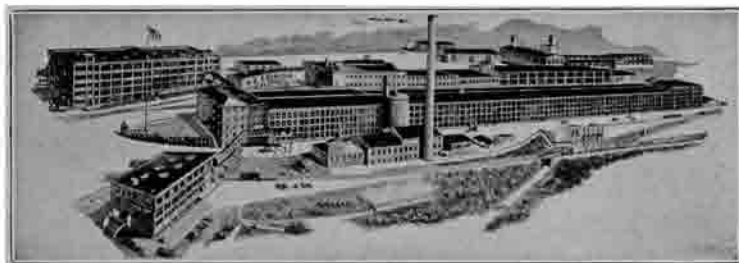
A Modern Industrial Plant
