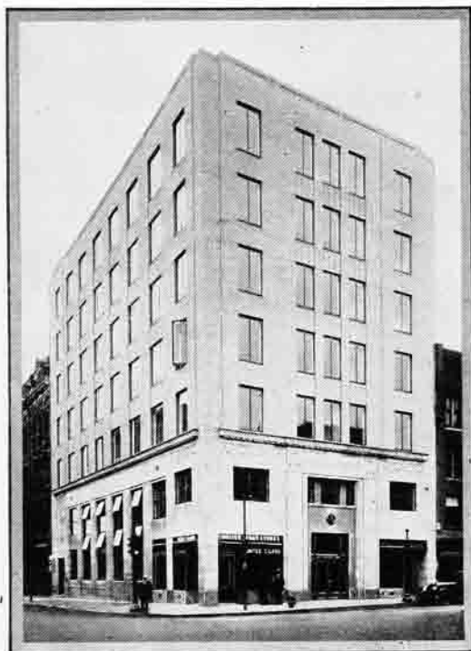
FIRST NATIONAL BANK BUILDING ERECTED
