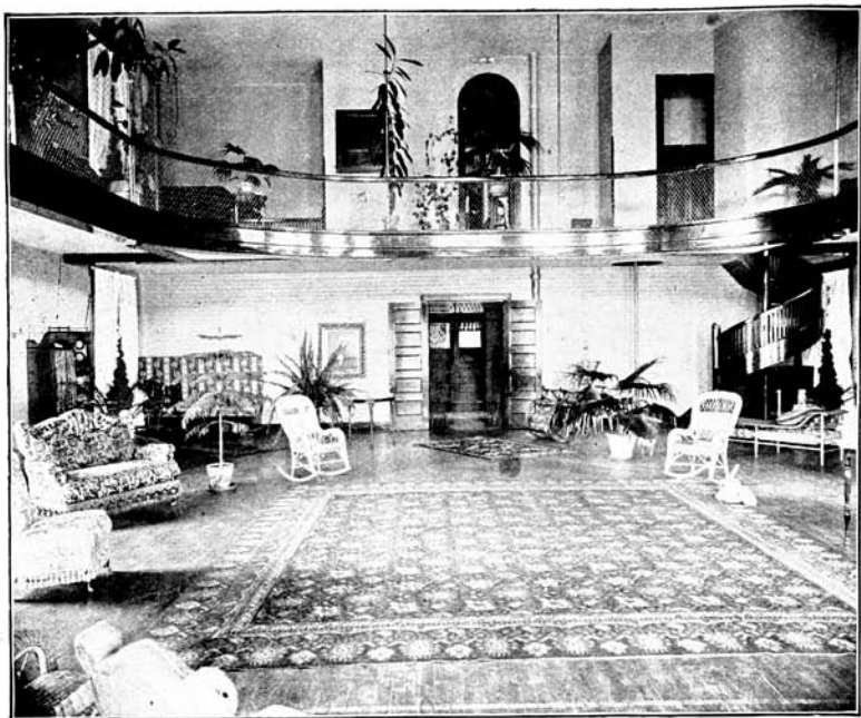
Gymnasium and romp room in the Pratt Private Hospital. - Front view.
