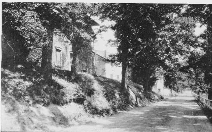
Old Wine Cellar on Hammondsport Street
