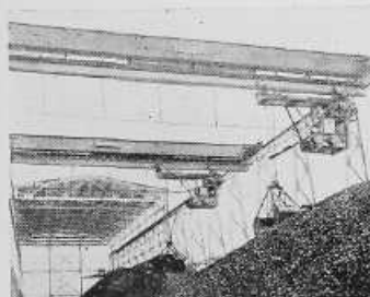
Transfer Cranes utilizing either floor or cage operated Shepard Hoists—the "Aerial Railway of Industry."
