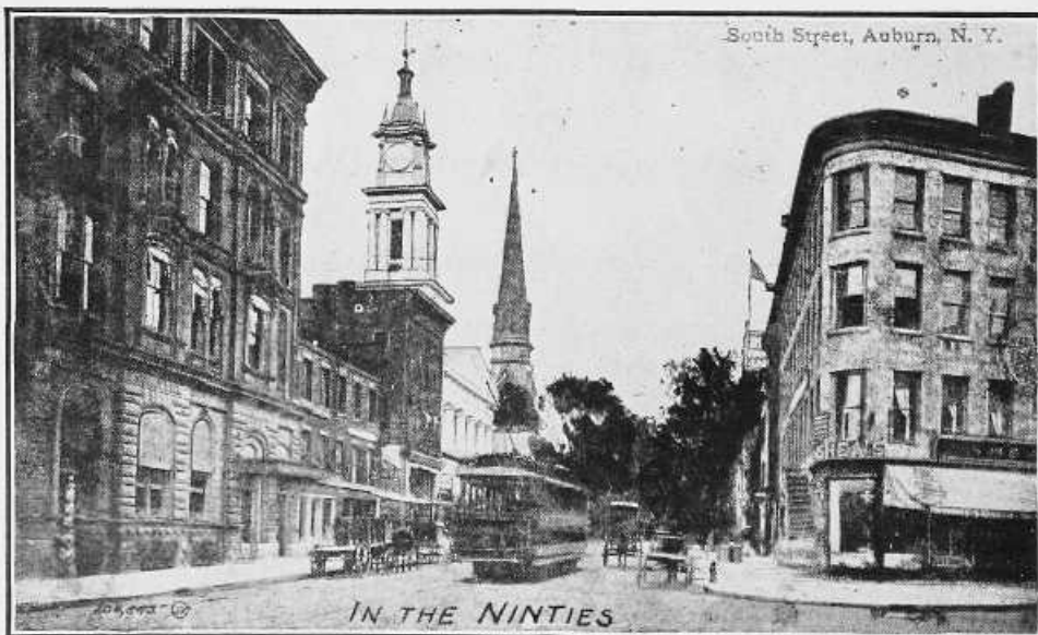
In the above picture are shown at the left, first the now abandoned Second Presbyterian Church, and farther in the distance the Universalist Church, Auburn. Both are still standing, excellent examples of old time church architecture.
