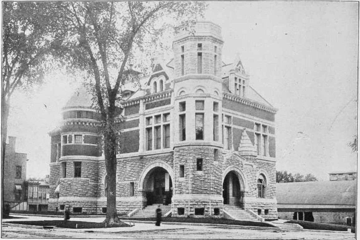
Post Office, Auburn, N. Y.
