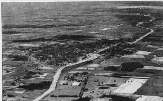
Tuttle & Nester Photo Waterloo and Seneca Falls along Greater Broadway as seen from the air
