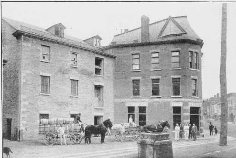
Stone mill, at Auburn, one of the oldest structures along the Genesee turnpike. It was erected more than a century ago by John Hardenbergh. The stone relic stands today.
