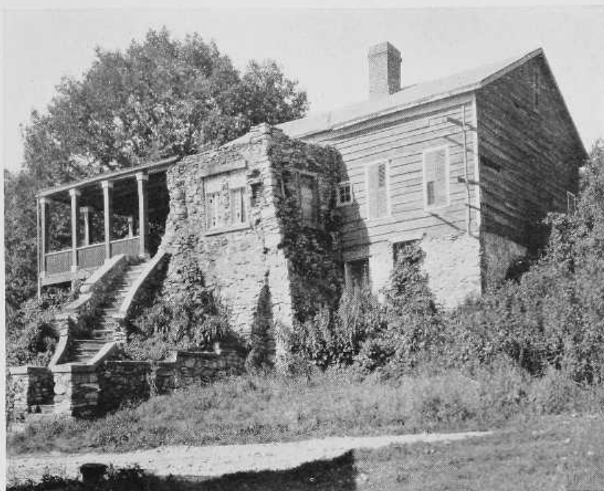
Remnants of the old toll gate office of the Cayuga Bridge at the Bridgeport end. The structure, now remodeled into a summer camp, was the residence of the toll gatherers. The front of the building and the north end have never been materially changed with the exception of slight repairs.
